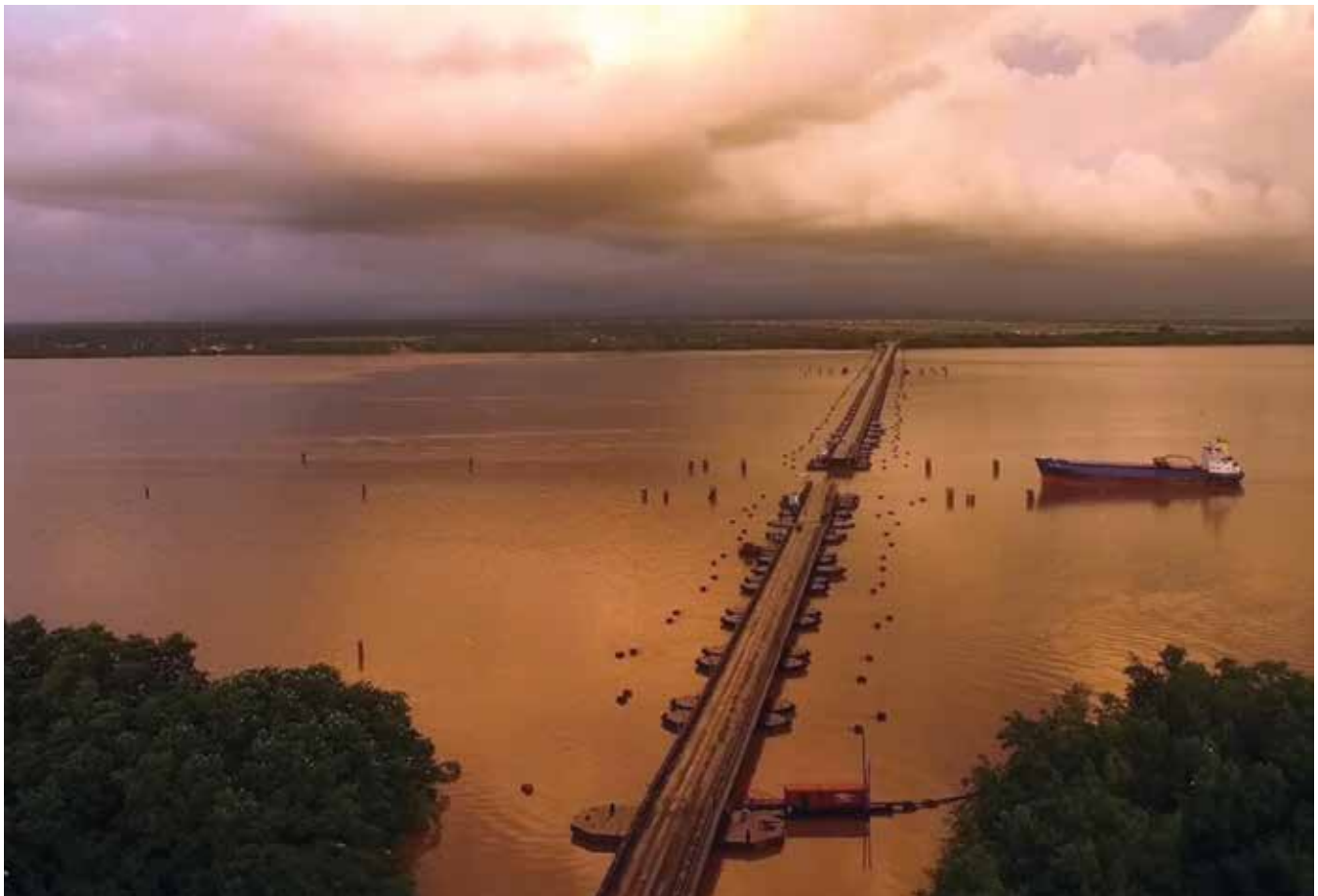
Demerara Harbour Bridge
